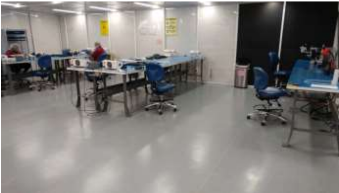
Standard VCT covered with the URAS / Titanium ESD Sheet Vinyl Flooring System. Easily Compliant to the latest ANSI ESD S20.20 standards
