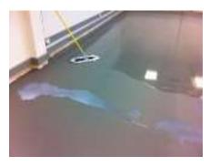
ElectraBond is used as an intermediate barrier coat between the first coat of cured ElectraGuard ESD Epoxy and the second coat of the epoxy. ElectraBond is used to extend the coverage of the more expensive epoxy and also hide imperfections in the concrete from repairs and variances in concrete texture.
