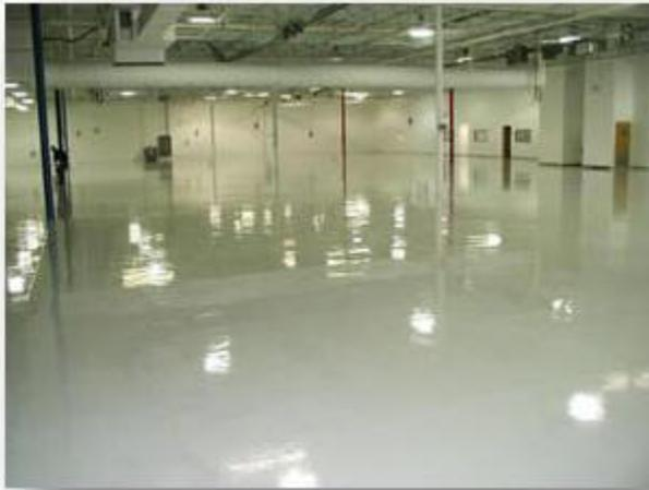
The ElectraGuard ESD Epoxy Flooring System meets the latest ANSI ESD S 20.20-2014 standards. It's warranted for life time static conductivity and features a 10 year life expectancy. ElectraGuard installations are seamless (with proper preparation of the concrete). ElectraGuard handles heavy loads and is resistant to high concrete vapor emissions (the number one cause of ESD Tile and thick set epoxy failures). ElectraGuard is made in the U.S.A! Unlike mere latex or other one part epoxy
