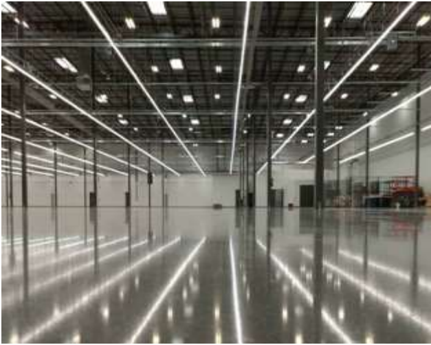
ElectraSeal Over Diamond Polished Concrete
