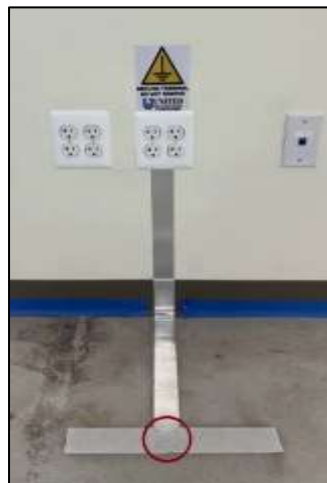
Figure 4, Completed showing center punched area
